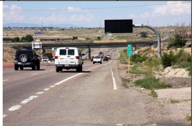
Figure 20. MP 313.0. No bedrock is present within survey corridor from this point east to eastern terminus of survey corridor. Photo view UTM 13S, 530895 mE, 4240517 mN (NAD83).
