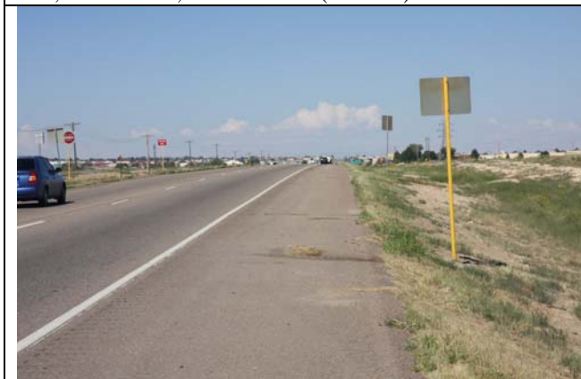
Figure 5. MP 311.0. View west northwest along westbound lanes of US 50 in area mapped as Slocum Alluvium. Lower limestone unit of Smoky Hill Shale Member was mapped just to the west of this area by Scott (1969), but was not observed in the field and may be located outside of the corridor . Photo view UTM 13S, 527921 mE, 4241192 mN (NAD83).
